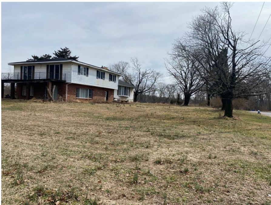
Photo 2: View of existing structure on the site.
