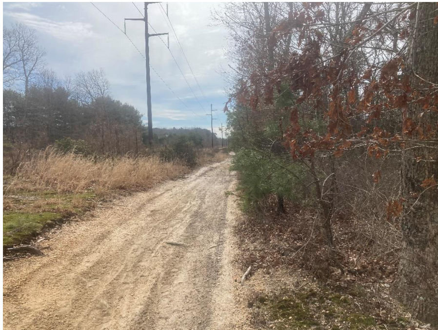
Photo 4: View of the access road and utility line within the northern portion of the site.
