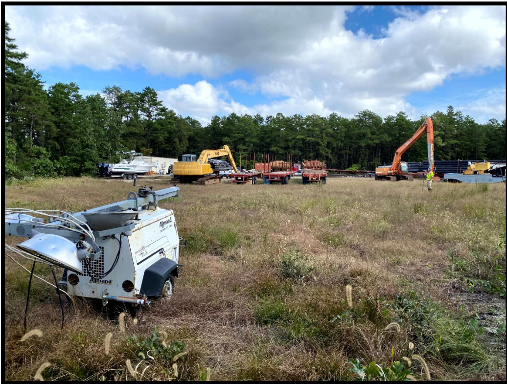
Photograph 6 – View northeast of the area where the pre-fabricated building is proposed.
