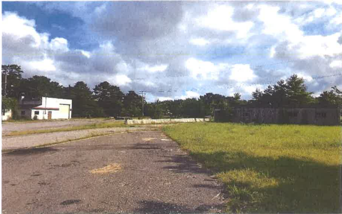
Photograph 5: View of the abandoned commercial structures within the southern portion of the site
